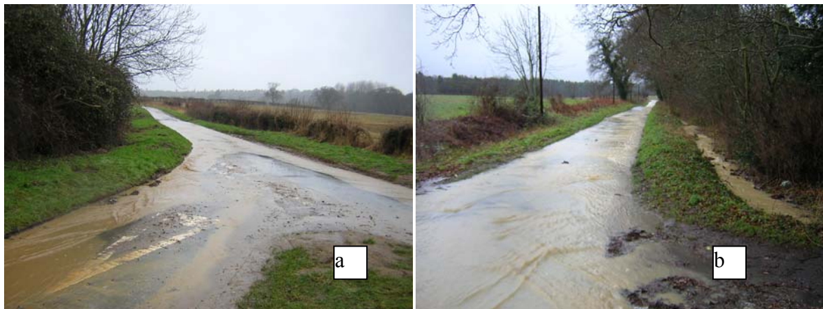
Figure 5.6 Fine sediment runoff from arable fields and road side verges. Note routeway into road side drain. Photo a) Gateley, TF972248. Photo b) Guist Bottom, TF987267.
