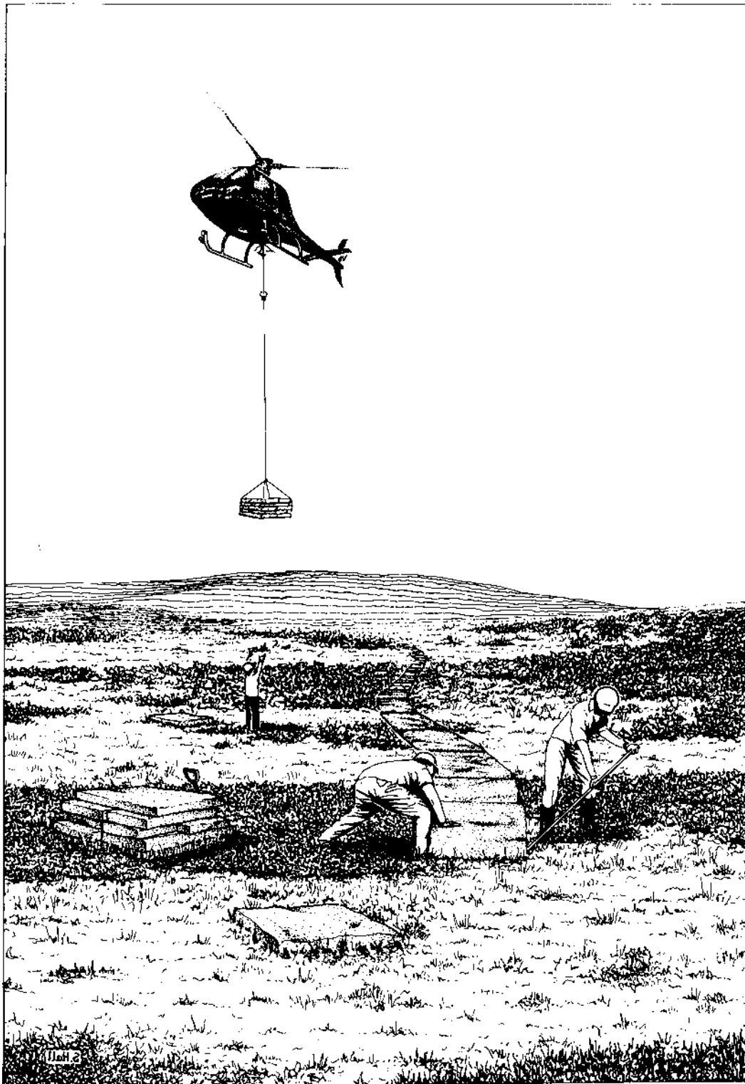
Figure 5.2. Stone flags have been used to surface footpaths over peat in montane areas in the North Pennines and Cheviot Hills. The material used for the flags should be compatible with the geology of the area. The flags float on the peat surface and provide a smooth walking surface. They allow re-vegetation of the surrounding bare peat and the edges and joints also grow over to make the path less obvious (see Information Note 10).
