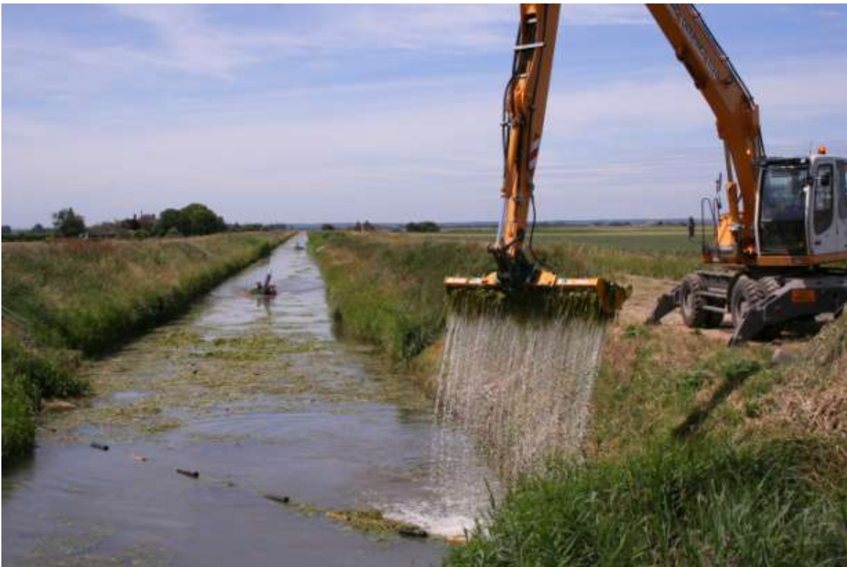
Plate 14 Weed-cutting in the Counter Drain at Pode Hole (8 th July 2010)
