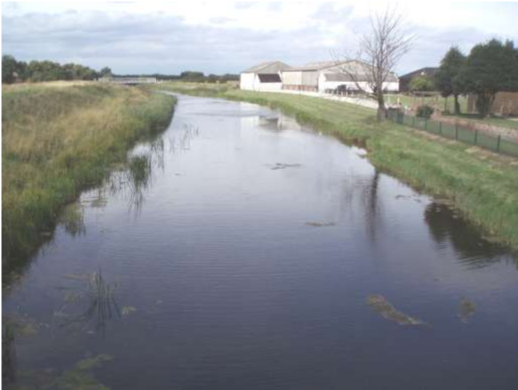
Plate 10 Vernatt's Drain section I near Spalding Hospital
