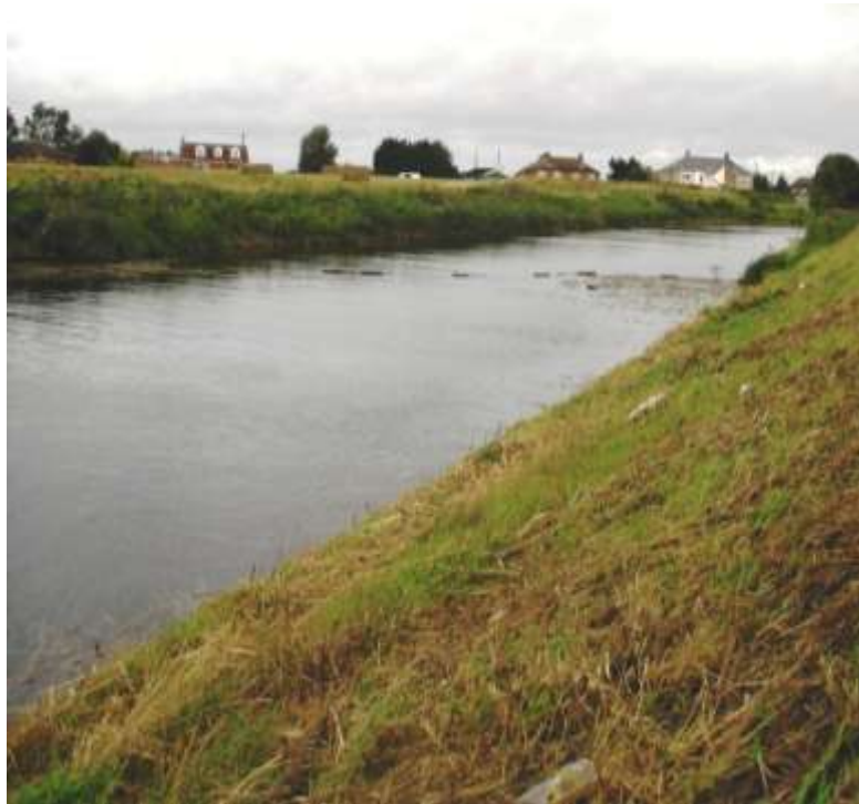
Plate 12 The South Drove Drain showing a boom installed to collect cut vegetation
