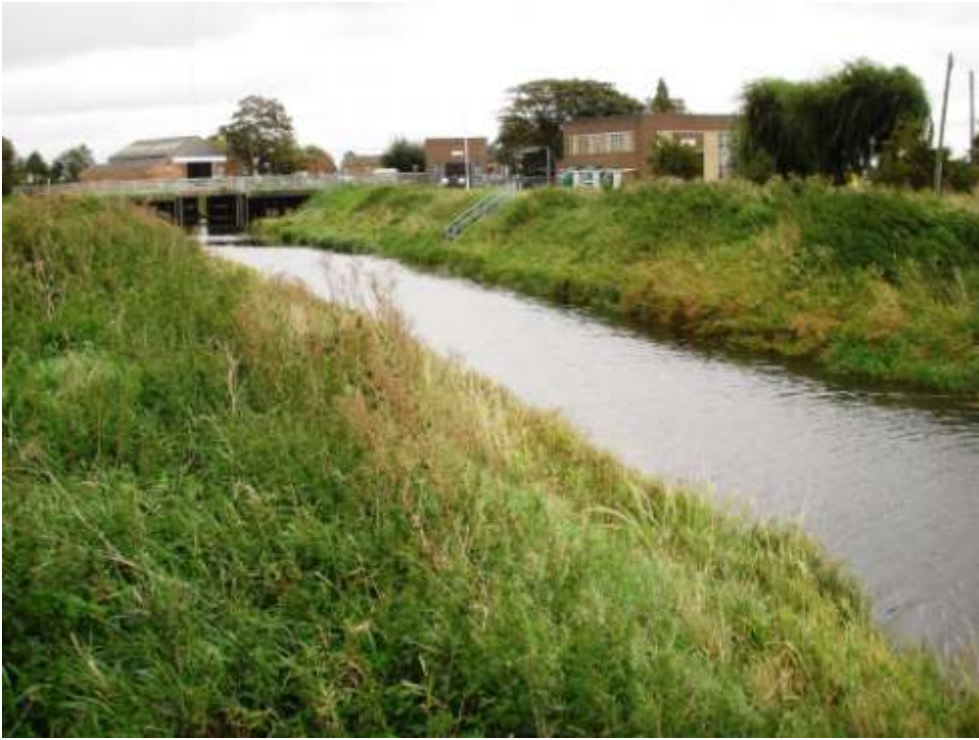
Plate 13 The gates at the upstream end of the pump basin on the Counter Drain at Pode Hole
