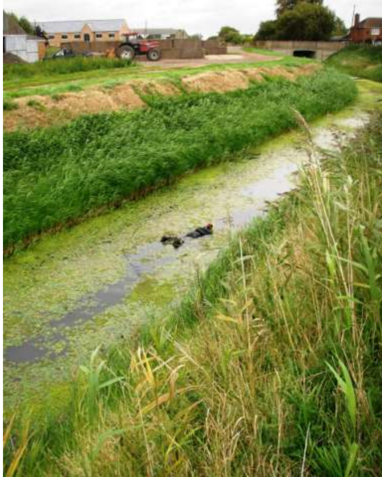
Plate 18 Surveying the Fourth District Main Drain at Pode Hole
