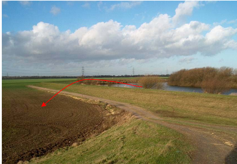
Figure A4.2 Flood storage area starts to fill by natural overtopping of flood banks.
