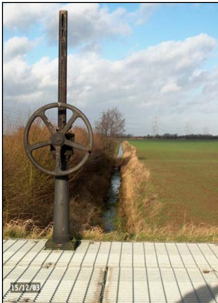
Figure 2.5 Controlled inlet. Saundby Beck (Beckingham Marsh) (Photo T.M. Hess)
