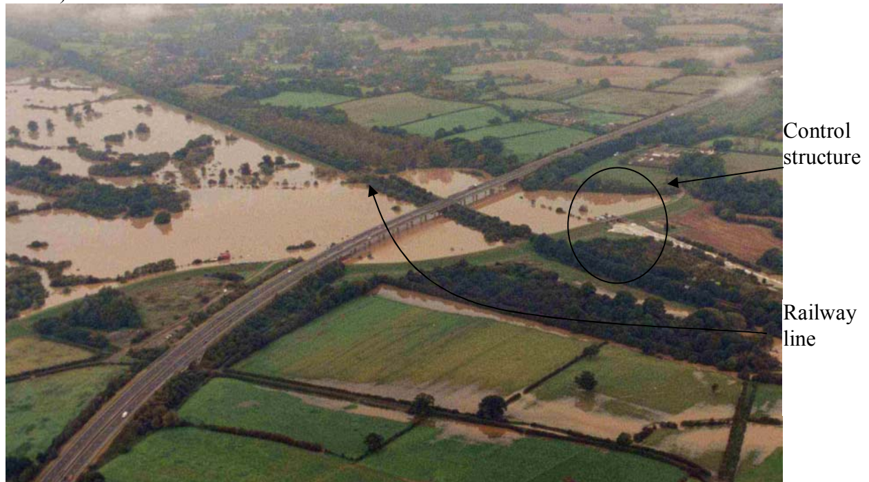
Figure A4.25 The Barrier in action during the 2000 floods. The road bridge and railway embankment can be clearly seen.
