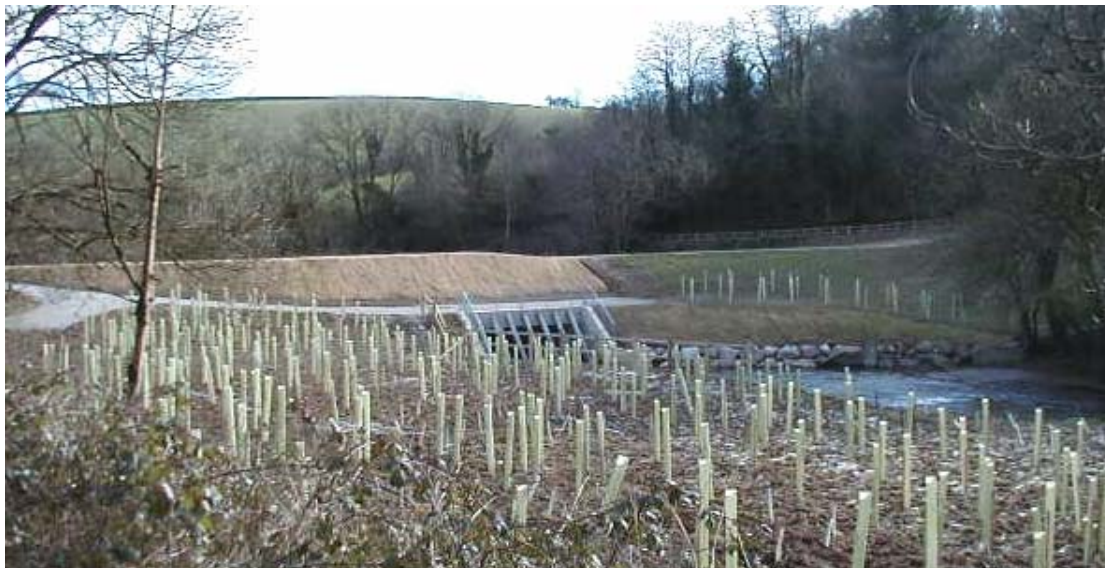
Figure A4.23 The dam and adjacent vegetation is designed to suit the surrounding landscape.
