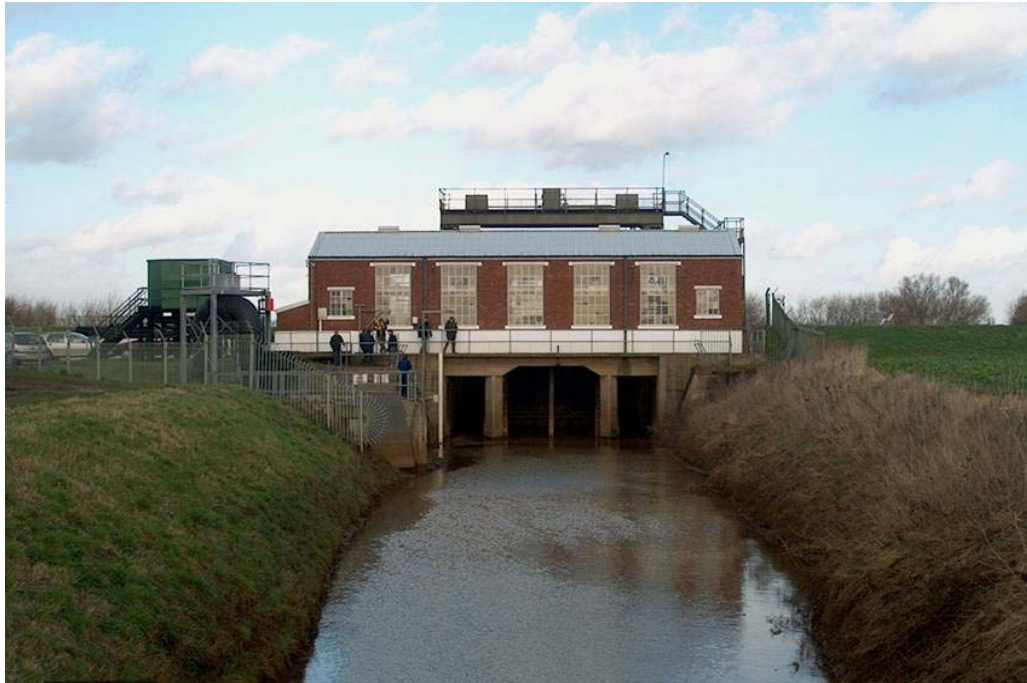
Figure A4.4. Beckingham Pumping Station is the only outlet for flood storage. A large sluice gate (centre) allows gravity drainage when the Trent is low. Otherwise pumps are used to lift water into the Trent.
