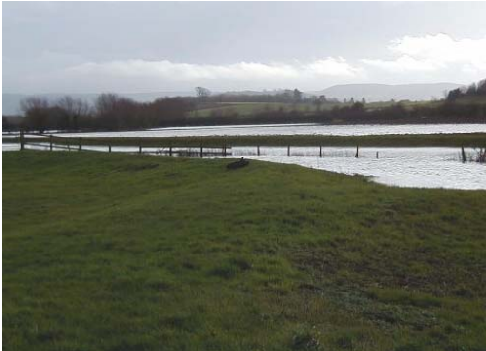
Figure A4.6. Coombe Hill washland storing water (background) with low flood banks of the River Chelt in the foreground.
