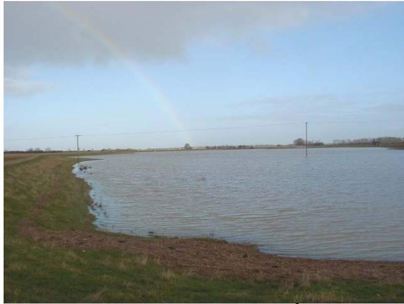
Figure A4.12 Manby washland in flood nearing its 18,300m 3 limit, note setback embankment on the left.
