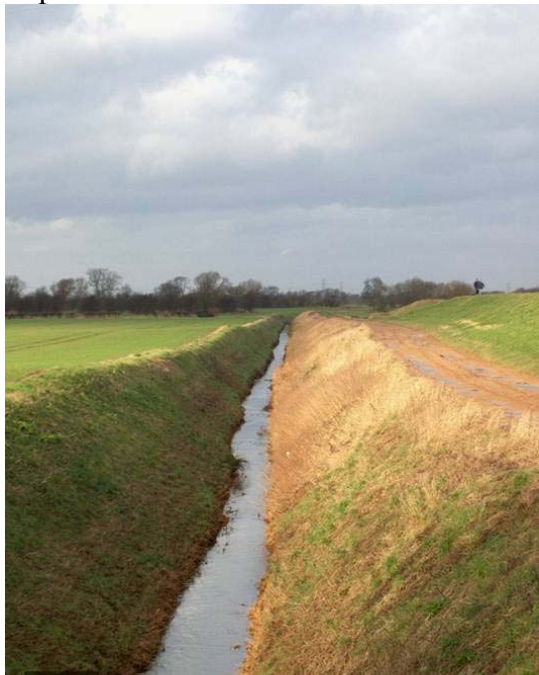
Figure A4.3. Main drainage ditch leading to pumping station.
