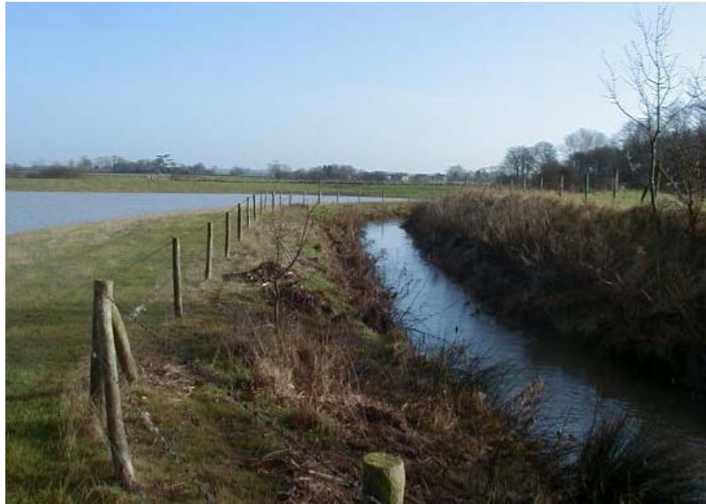
Figure A4.15 Long Eau flanked by old engineered bank (right) and the lowered re-profiled bank (left).
