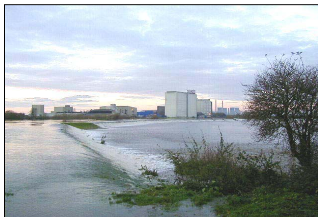
Figure 2.4 River Trent overtopping flood banks at Beckingham Marshes, Gainsborough
