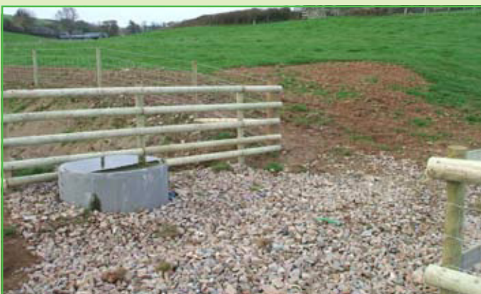
Culvert, cattle crossing, drinking point
