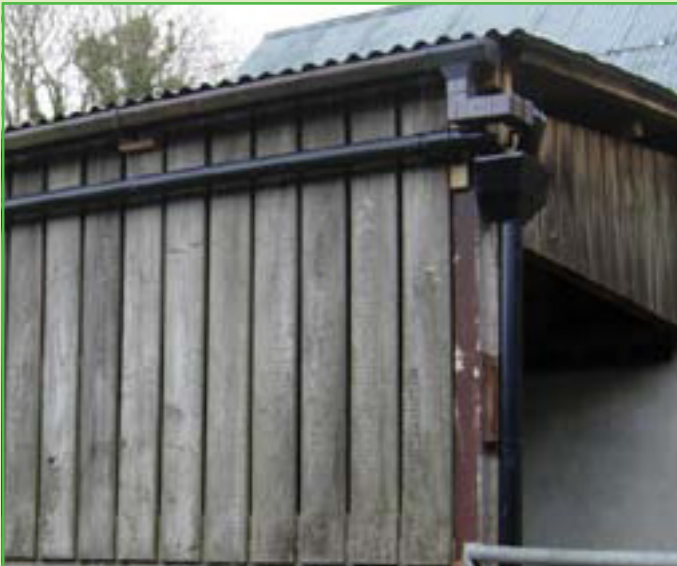
Newly guttered roof
