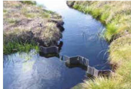
Figure 14. Plastic piling in gully on blanket bog, good water table elevation. Peak District. Water flows from top centre down the photograph to bottom left in a small gully on fairly flat ground. Note the overflow lip in the centre of the dam (Photo: Penny Anderson)
