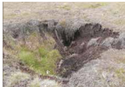
Figure 9. Peat pipes form from underground drainage, collapsing to form more gullies and 'swallow holes' (Photo: Penny Anderson; Peak District)
