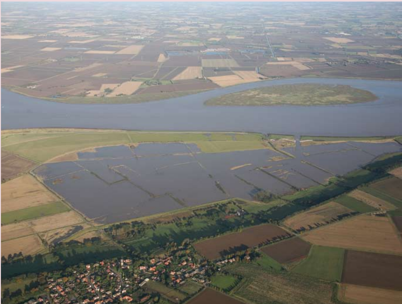
Alkborough Flats inundated following a breach in the flood defence bank
