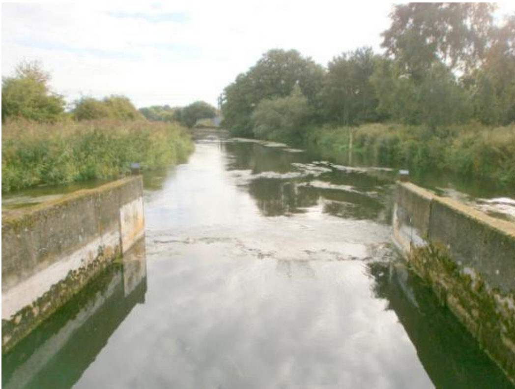
Figure 8. Upstream of Ringwood Weir.
