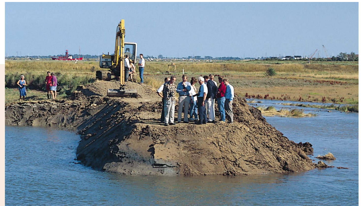
Managed retreat breach point on day one - high tide. Tollesbury, Essex. Peter Wakely/English Nature 19,856
