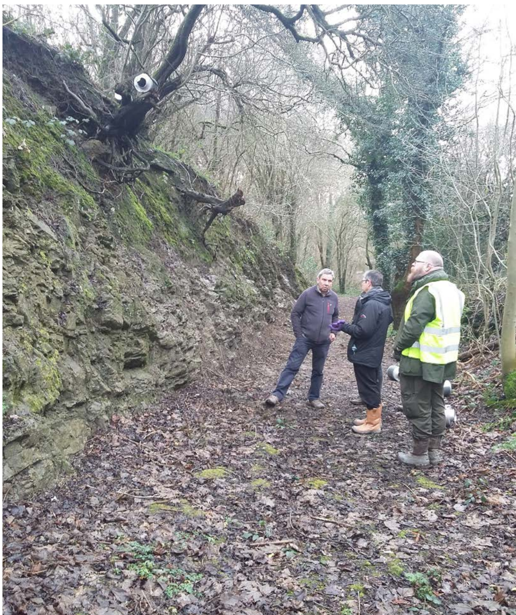
Wagon-way, January 2018. Faces cleared of scree, vegetation and soil adhering to face and in cracks. ©Natural England/Jonathan Larwood
