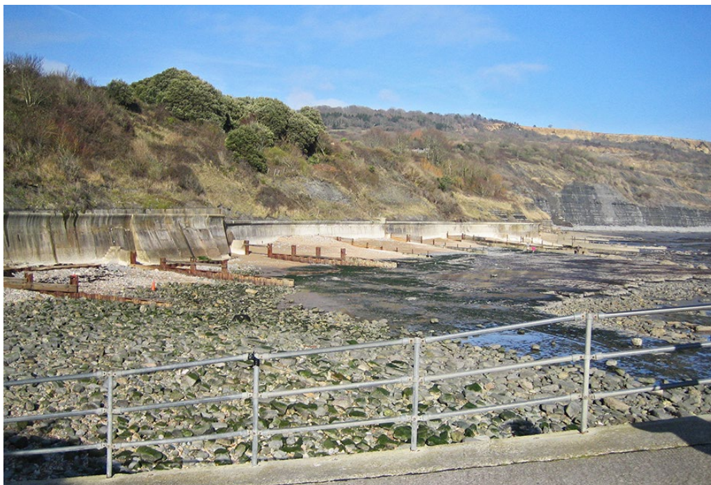
Church Cliff and East Cliff in 2008. In the distance, the Spittles landslide consisting of mudstones belonging to the Charmouth Mudstone Formation with its back scar in the Upper Greensand. Foreshore of ledges in the Blue Lias Formation with a failed groyne-field. Cliffs in the Blue Lias Formation obscured by scoured and corroding seawall, with unstable slopes above. ©Natural England/Dave Evans
