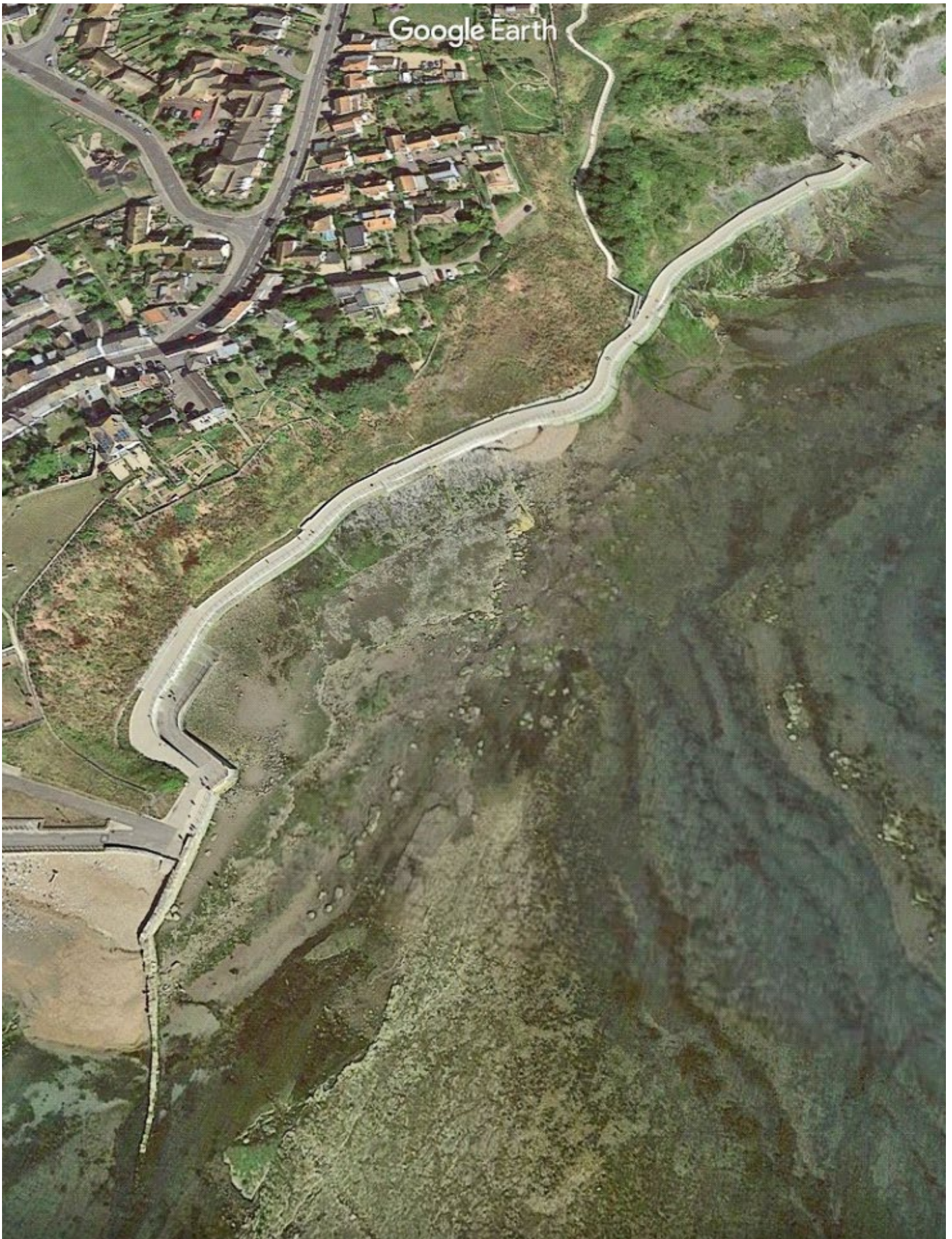
Google Earth image of completed scheme with access route on the top of the seawall together with access ramps onto the foreshore. Exposures of the upper part of the Blue Lias Formation within reach from the access on the seawall. Path leading from carpark down to seawall acts as pedestrian access into the centre of Lyme Regis and also marks the eastern limit of the stabilisation works on the upper slopes. ©Google Earth visited 2018. Imagery Date 8/15/16.
