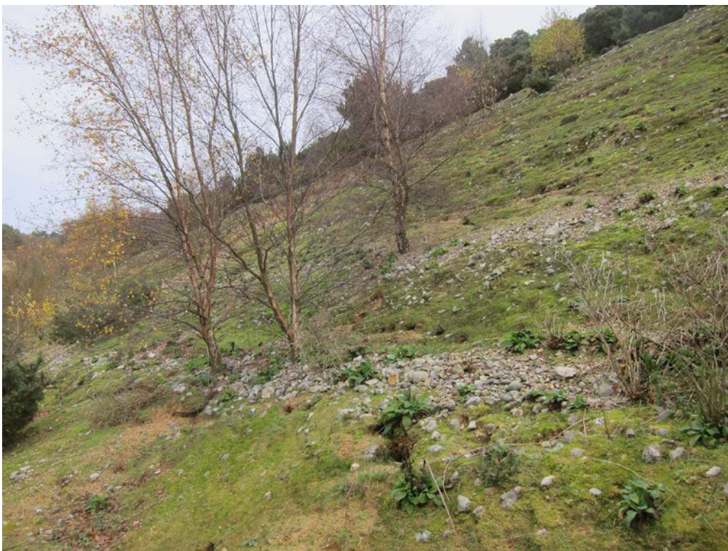
Face on eastern side of the southern part of Briton's Lane Quarry SSSI, Norfolk. These steep and high slopes have no permanent exposures and are being allowed to revert to heathland. The slopes form from bench failure, so that much of the original face is covered in a layer of talus that varies in thickness across each of the original benches. ©Natural England/Dave Evans
