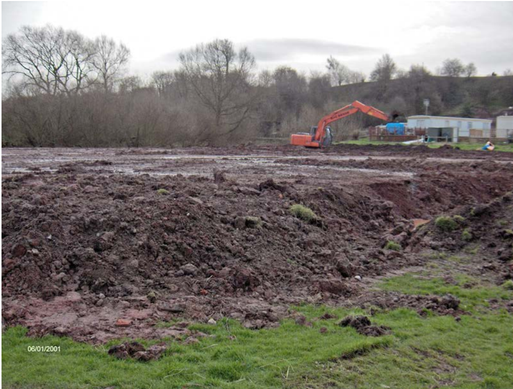
Raising and levelling of land forming part of the River Dane flood plain as a flood defence and for the extension of the caravan site. ©Natural England/Anna Wetherell
