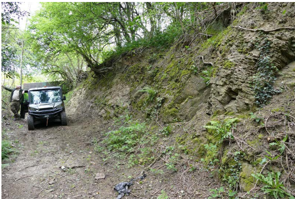
Wagon-way section, January 2018. During clearance – all terrain vehicle in floor of cutting with exposures of the Upper Whitecliffe Formation and the base of the Downton Castle Sandstone Formation exposed in the cutting. ©Dudley Metropolitan Borough/Graham Worton reproduced with permission
