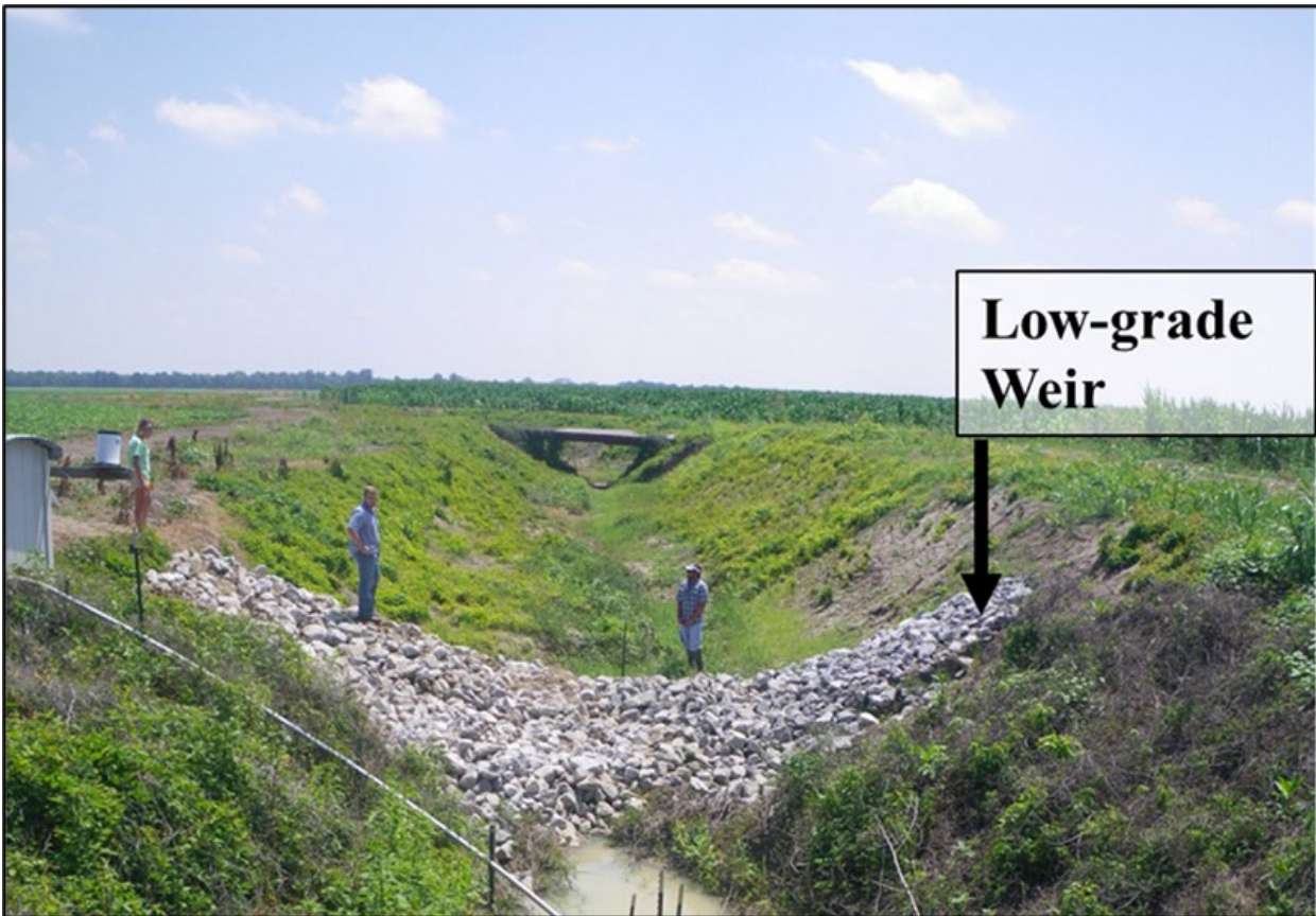
Figure 2: Example of a low-grade weir installed in a drainage ditch in Mississippi, USA. It is noted that the drainage ditch in this image considerably larger than drainage ditches typically seen in the UK. (Source: Kröger et al., 2011)
