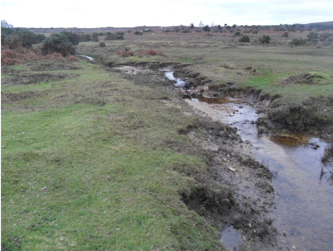
Figure 1-11: Knick point erosion on the tributary channels of Latchmore Brook.
