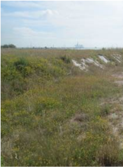
Photo 13 - partially vegetated ballast banks in C2
