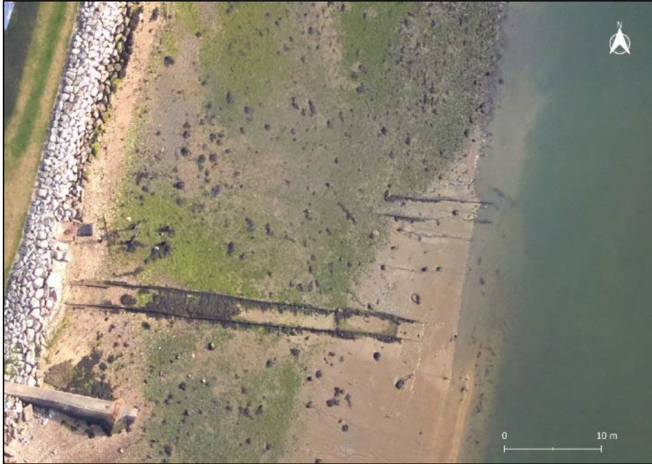
Figure 10. Abandoned structure with clear crossbeam support features.
