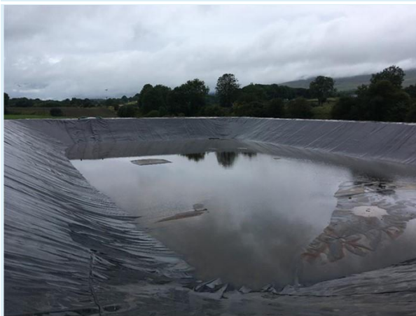
Floating slurry store cover © Natural England, Chris Turner
