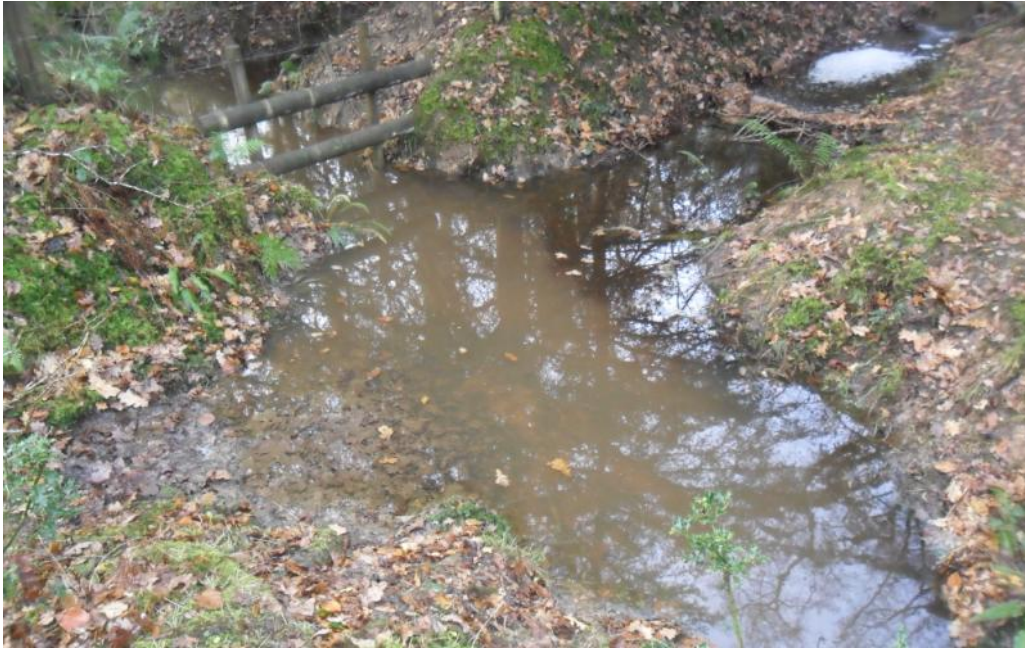
Figure 1-4: Silted drains entering the Avon Water
