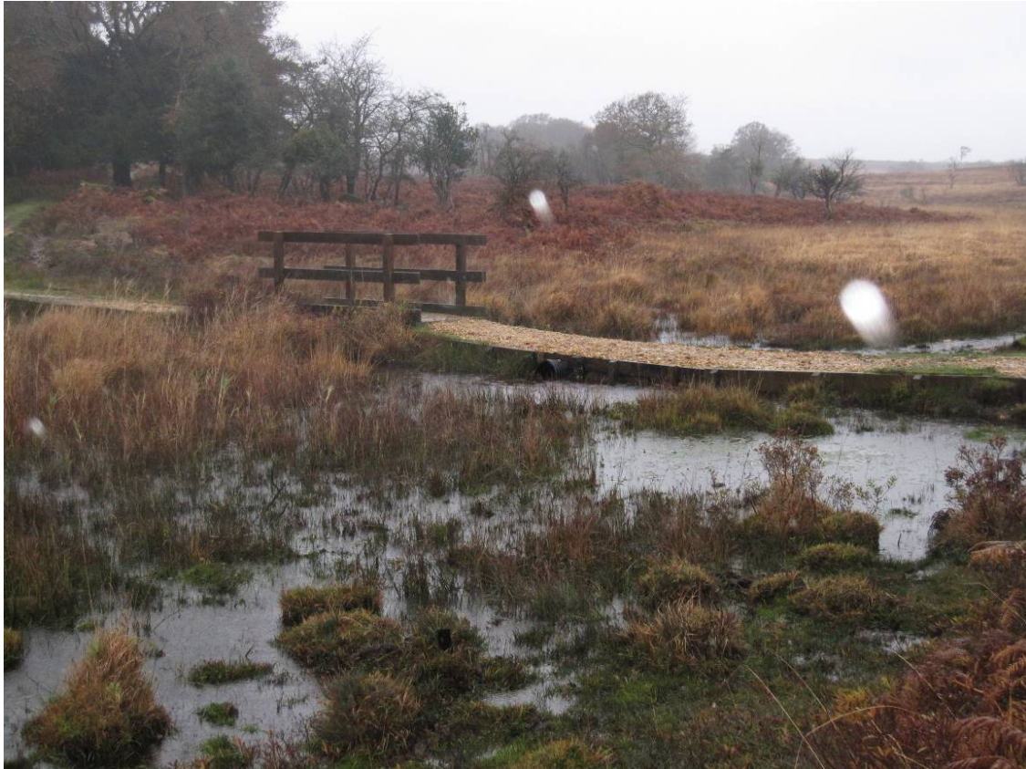
Figure 1-6: Ponding of water around footpath
