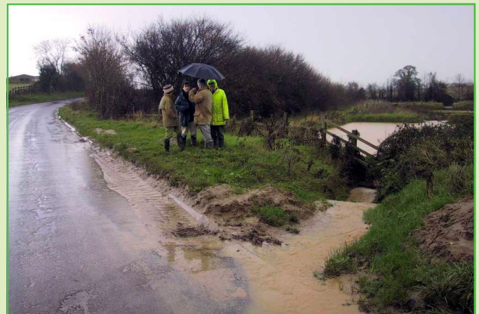
Run-off enters Highways balancing pond, site 2
