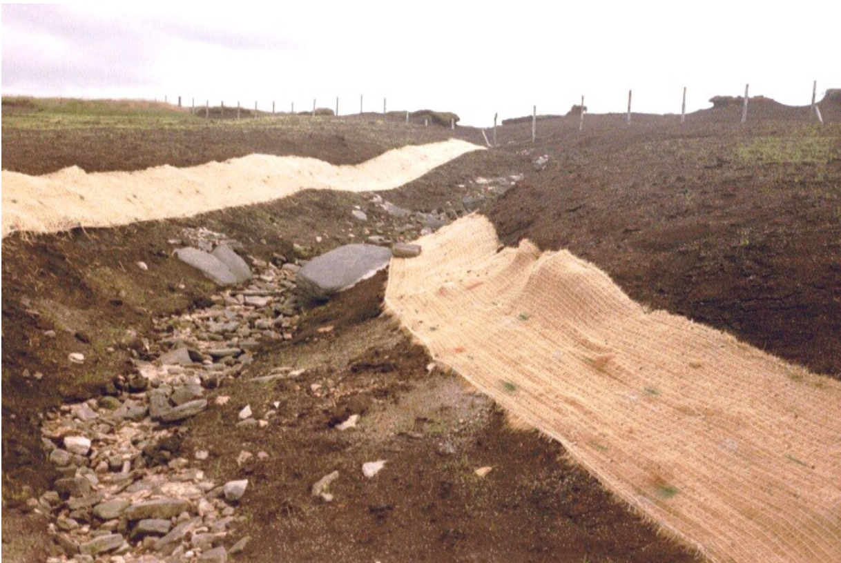
Plate 7 Geojute stabilising bare peat for moorland restoration project
