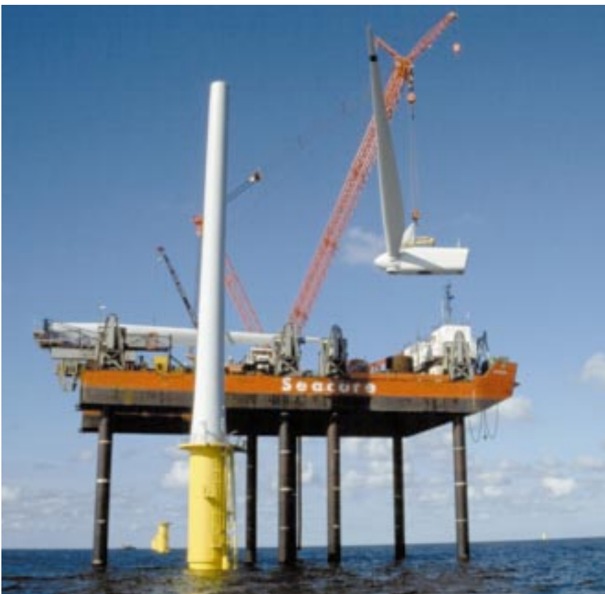
North Hoyle windfarm under construction. Martin Bailey/English Nature (above)
