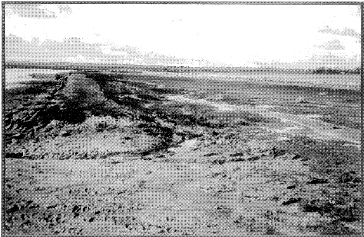
Photograph 2: February 1995 Looking from east to west across the spillway. This shows that the spillway channel has not yet become connected with the 'creek'.
