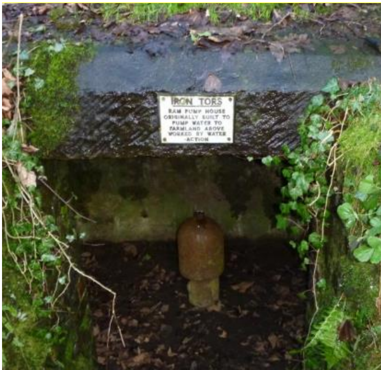
Figure 4 Photograph of Ram Pump.
