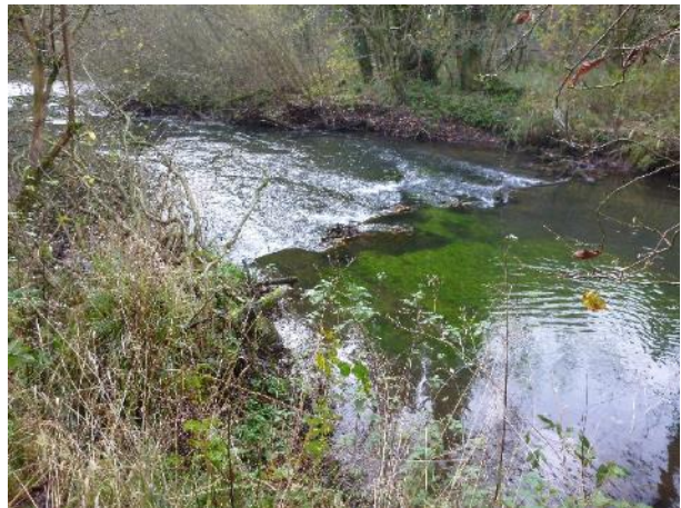
Typical weir in more confined section.
