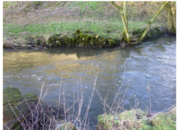
Example of stone bank protection typical of much of the river.
