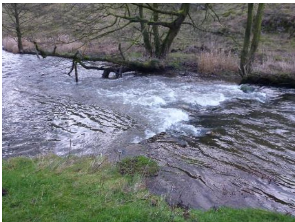
Weir beginning to break down.
