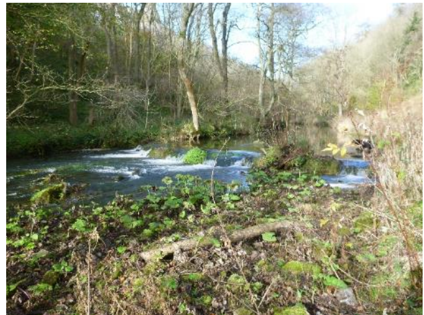
Weir built over natural boulders.
