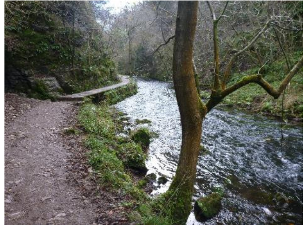
Causeway and associated bank reinforcement.
