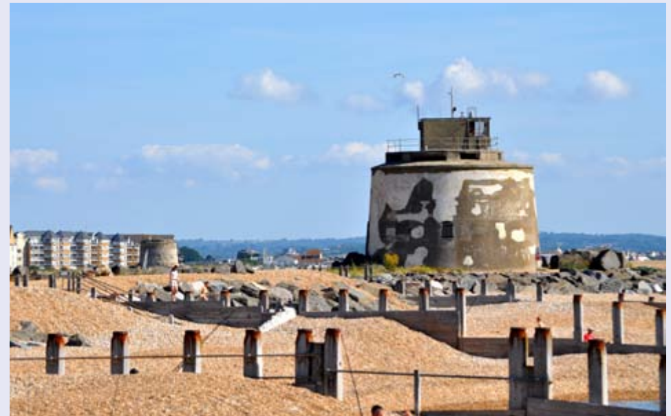
Martello towers on the shingle beach at the entrance to Sovereign Harbour. The High Weald is in the far distance.
