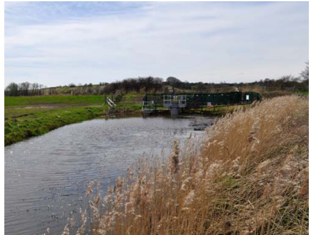
Water levels on Pevensey Levels are controlled by a series of pumps, sluices and other structures.
