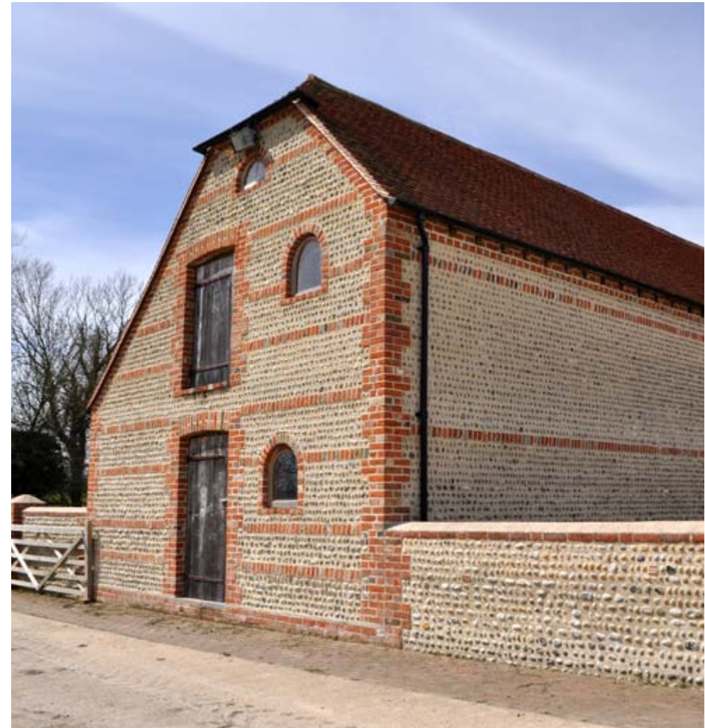
Sensitive restoration utilising traditional local building materials.
