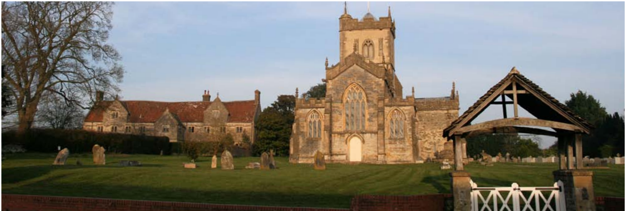
Most of the villages in the NCA feature a fine church and manor house. Here at Ditchat the two stand side-by-side. The church has been listed at grade I, while the Manor is grade II*
