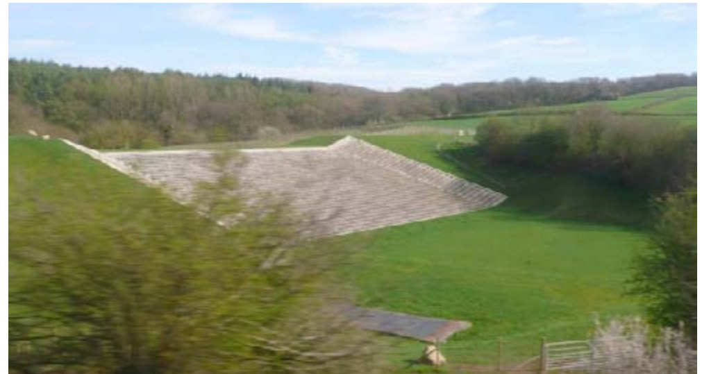
The ancient town of Bruton has been vulnerable to flash flooding due to its location, surrounded by steep hills with many small streams flowing off them. In order to protect the town from storm flows a flood storage reservoir and dam with spillway were constructed in 2008.
