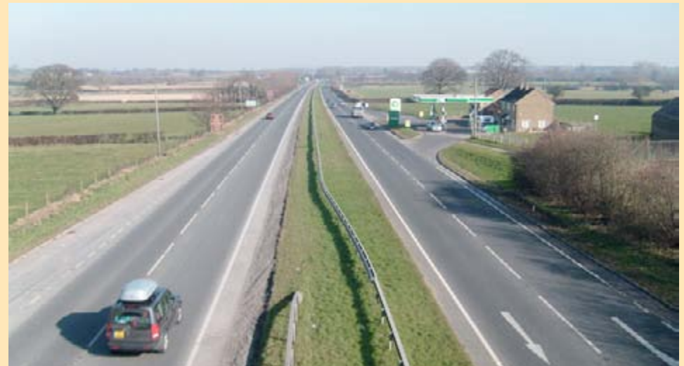
The A303 is a major trunk road that crosses the NCA east to west, duelled, as here, for much of its length it in places dominates the landscape but in more undulating areas can be happened upon quite suddenly.
