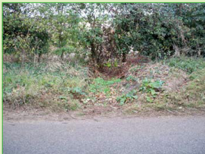
Cutting this gap in the hedge bank on the opposite side of the road from GCF should channel any running water into the grassland field corner beyond.
