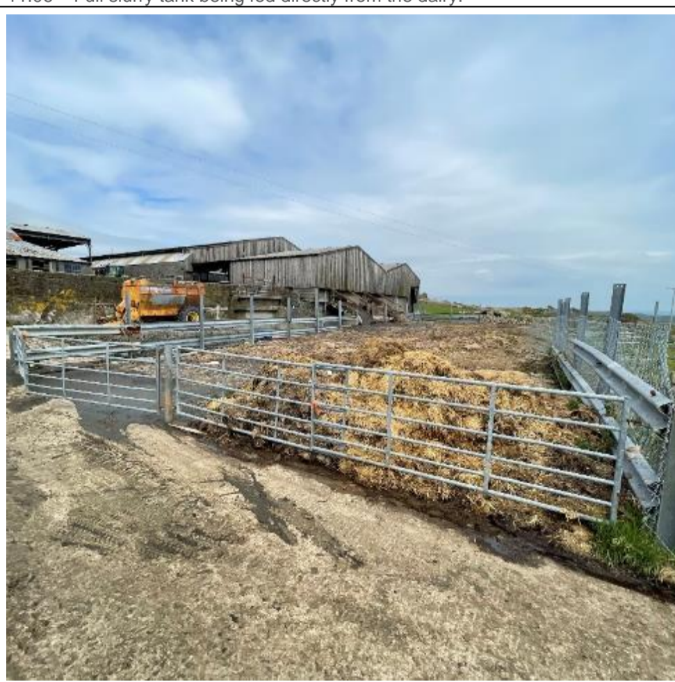
11.08 – Run-off from yard flowing towards fields.
