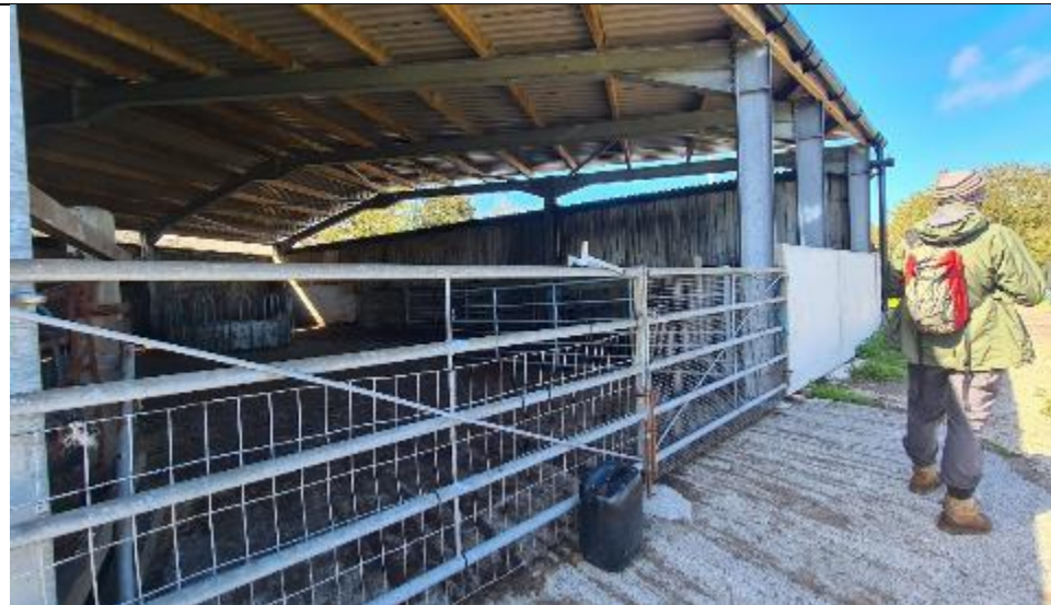
7.11 – Cattle handling facility.
