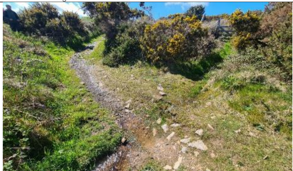
7.07 – Footpath as active flow pathway.
