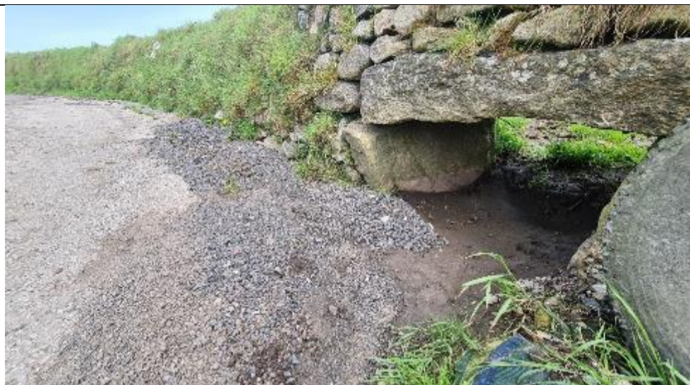
11.10 – Sediment deposited on path during rainfall events. Hole in field wall (filled with fine sediment) and sandbag in foreground used to direct water into field.
