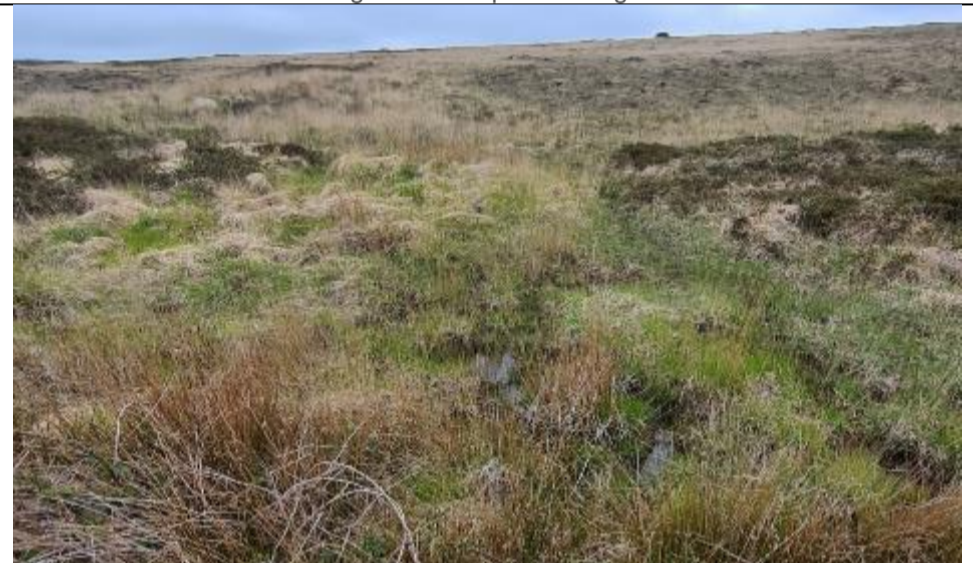
8.07 – Wet habitat upslope of road suggesting that road ditch may be blocked.
