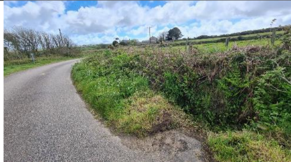
7.08 – Road verges cut to provide road drainage.
