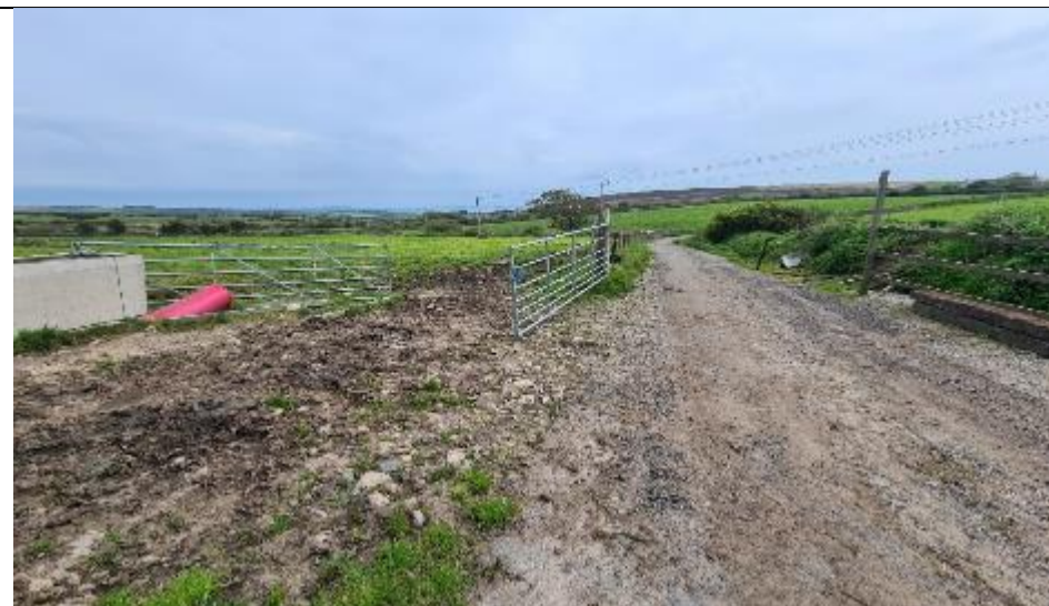
11.09 – Run-off along track leading from Middle Tregerest Farm.
