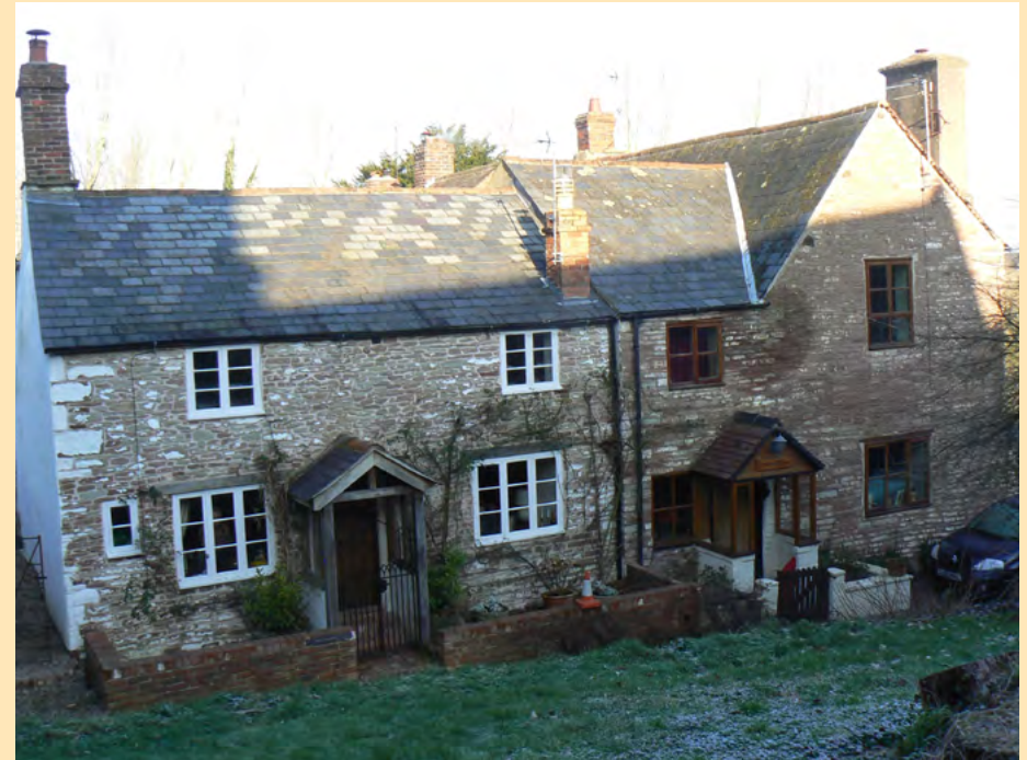
Listed buildings in Withington, built of local Withington stone, a distinctive pale greenish-grey Devonian sandstone once extensively quarried for local buildings in the village.
