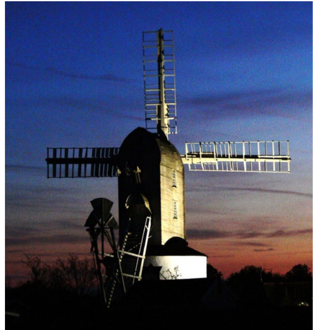
Saxtead Post Mill provides a strong sense of place and history, as seen here lit by the High Suffolk evening light.
