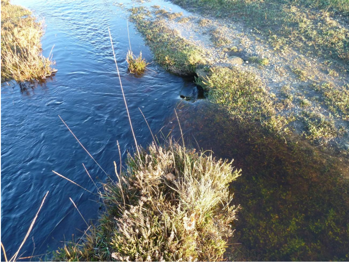
Figure 1-9: Pipe underneath road with grazed lawn (M23a) either side of it
