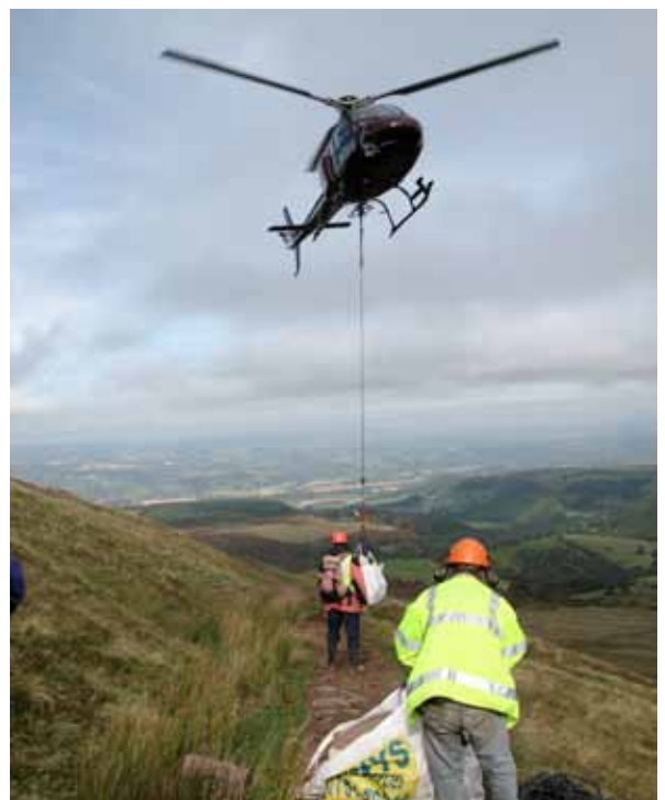
Stone Laying works on the Offa's Dyke Path.
