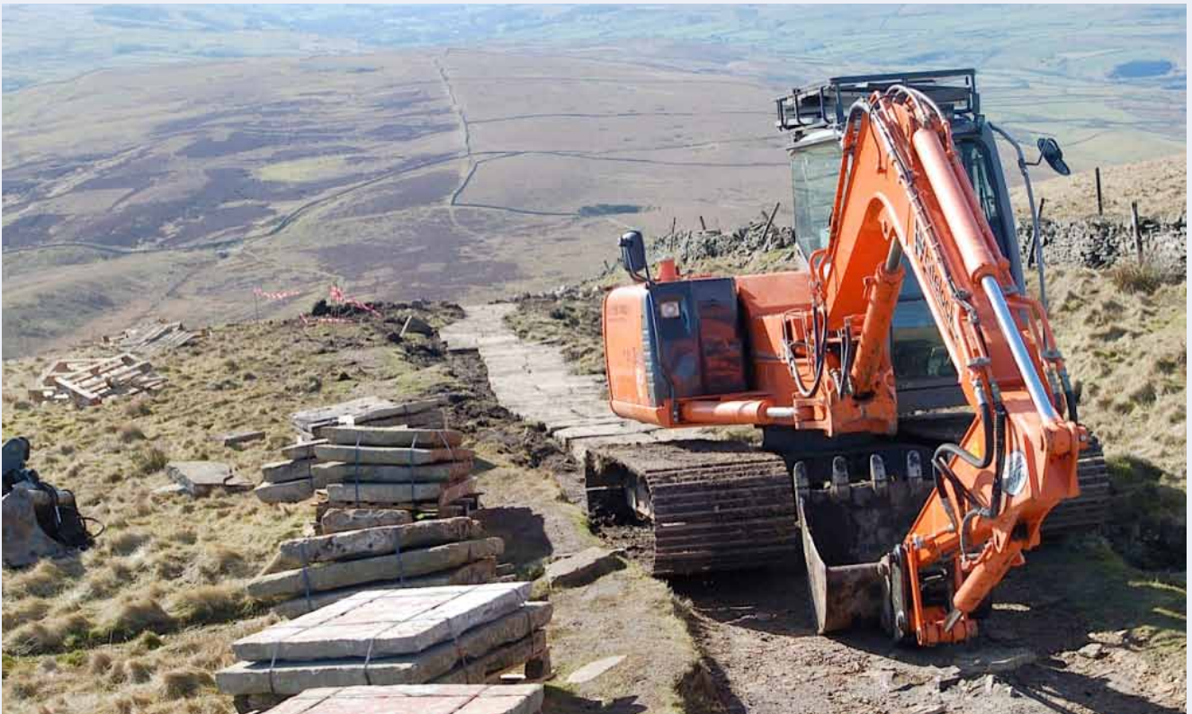
Flagstones being laid on Pen y Ghent.
