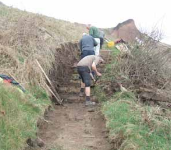
Skinningrove revetment and step work.
