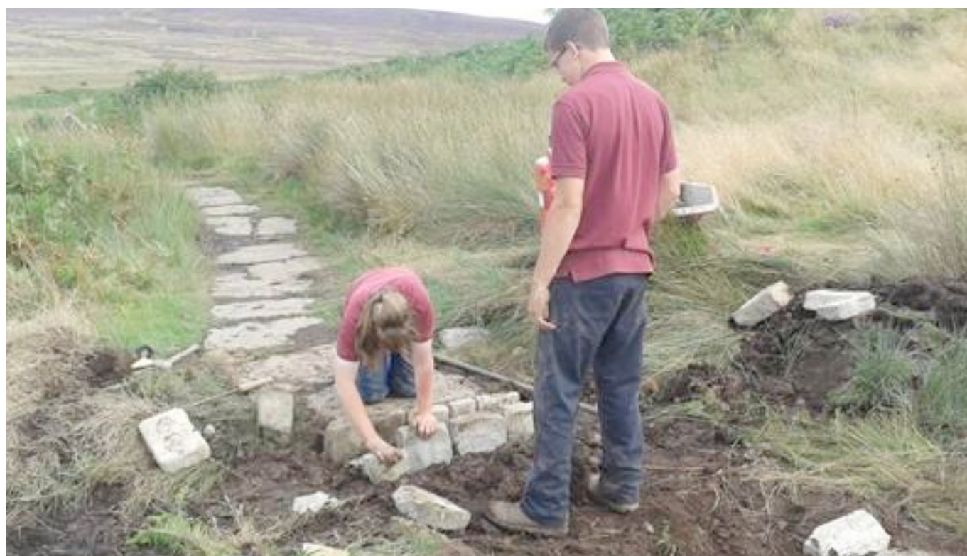
National Park apprentices slabbing and ‘pitching’ at Hutton Moor (Cleveland Way)
