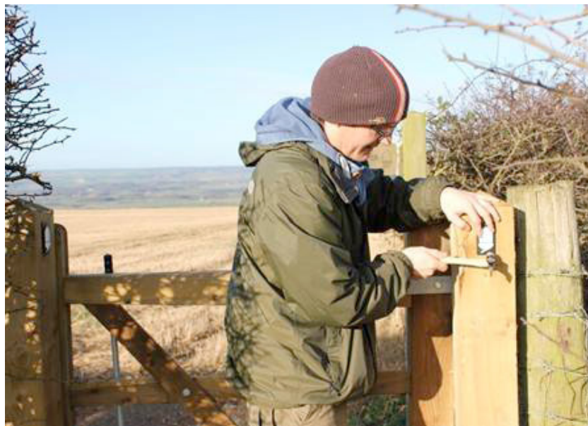
Completing access improvements on the Yorkshire Wolds Way
