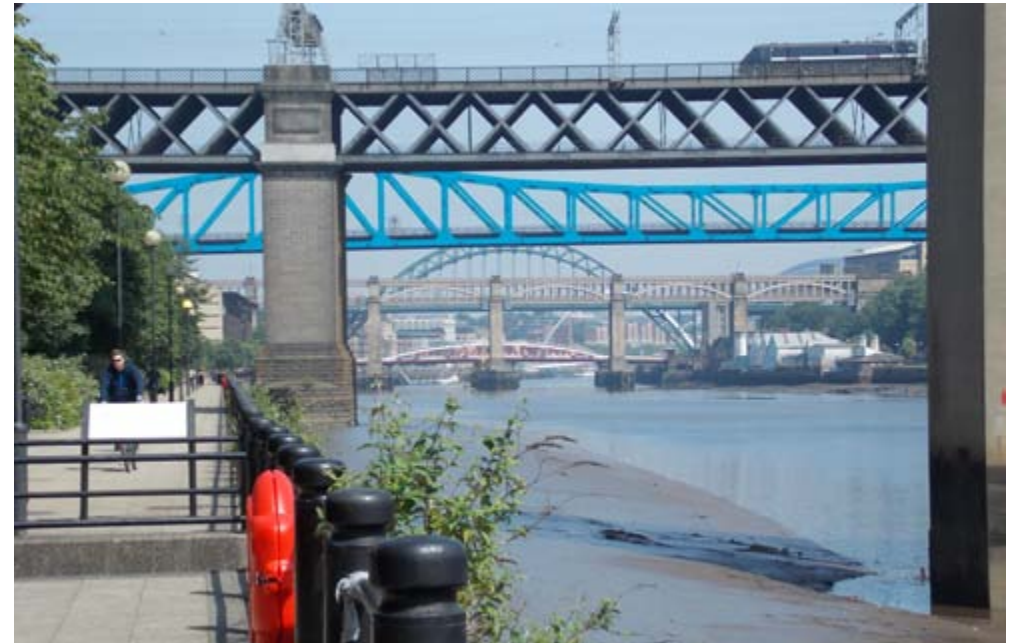
Dramatic bridges were built to link Newcastle and Gateshead across the Tyne.
