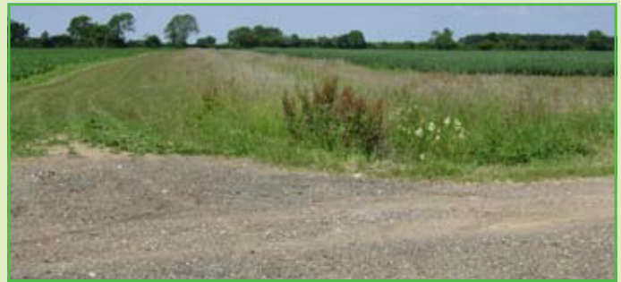
Use of road planings on track
