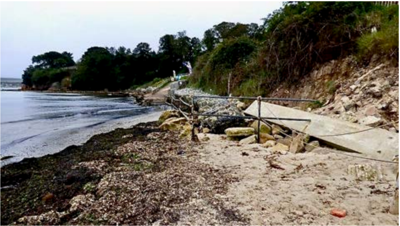
Fig. 8.10: Coastal erosion damage at Studland Beach in 2020. Ongoing erosion has led the National Trust to implement a policy of managed realignment at Studland. Courtesy: Sandy Gerrard/Creative Commons Licence.
