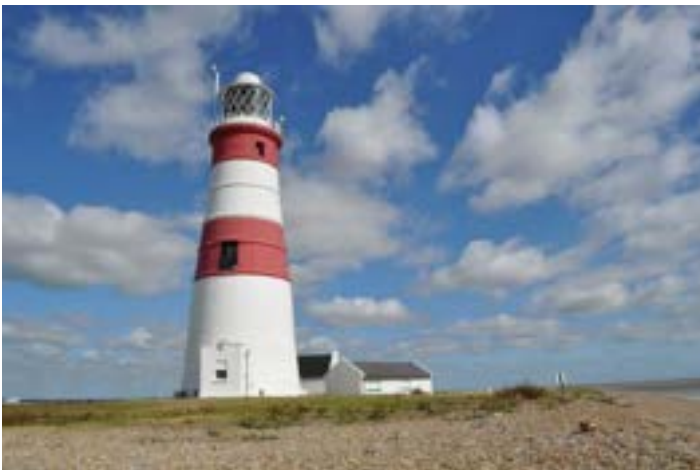
Fig. 3.18: Orford Ness Lighthouse; demolished in 2020. Courtesy: © Ashley Dace/Creative Commons Licence.
