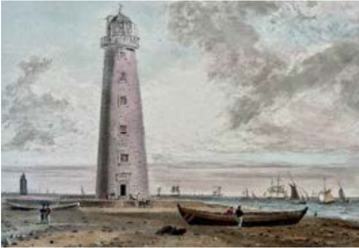
Fig. 3.17: This aquatint engraving by William Daniell shows the ‘Orford Ness Lighthouse’ in 1822, with its neighbour, the ‘Low Light’, about 1.5 km beyond. Daniell’s view shows a low shingle and sandy beach, with steps leading up to the entrance to the lighthouse. Comparison could be made with beach levels against the lighthouse structure until its demolition as a result of coastal erosion in 2020. Private collection.
