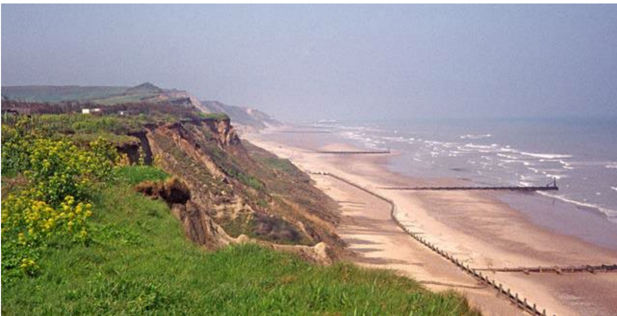
Fig. 2.12: This present-day photograph shows the cliffs looking from Overstrand towards Cromer. Although a timber breastwork fronts the cliffs, it is evident that instability processes are still active, thereby maintaining the cliff habitats. Courtesy: © Christine Matthews/Creative Commons Licence.
