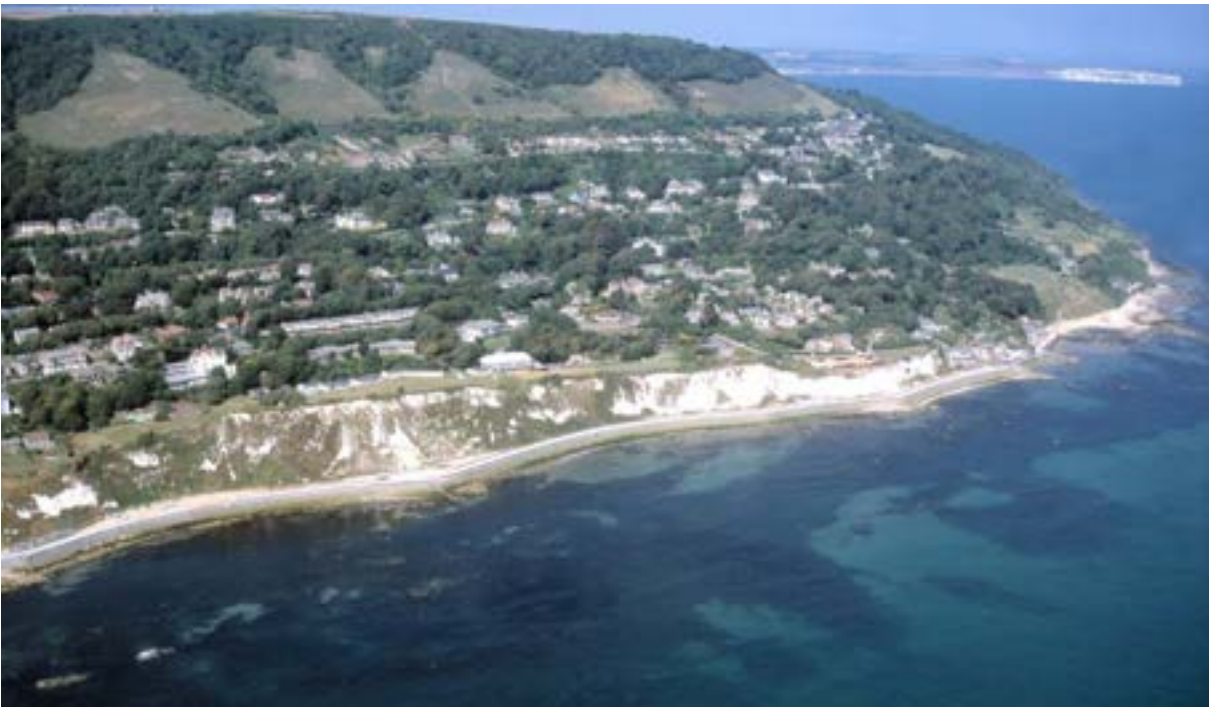
Fig. 7.21: The coastal frontage between Bonchurch and Ventnor is protected by a seawall for property and assets upslope. The photograph shows the seawall today. Courtesy: Andy Butler.
