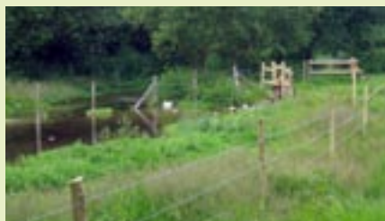
Figure 3. Drinking bay following fencing and pump installation
