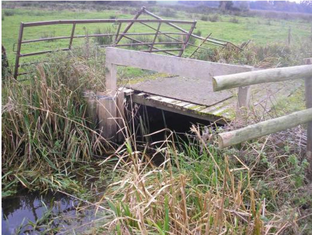
Figure 6.9. Unused hatch structure on Ibsley Stream.
