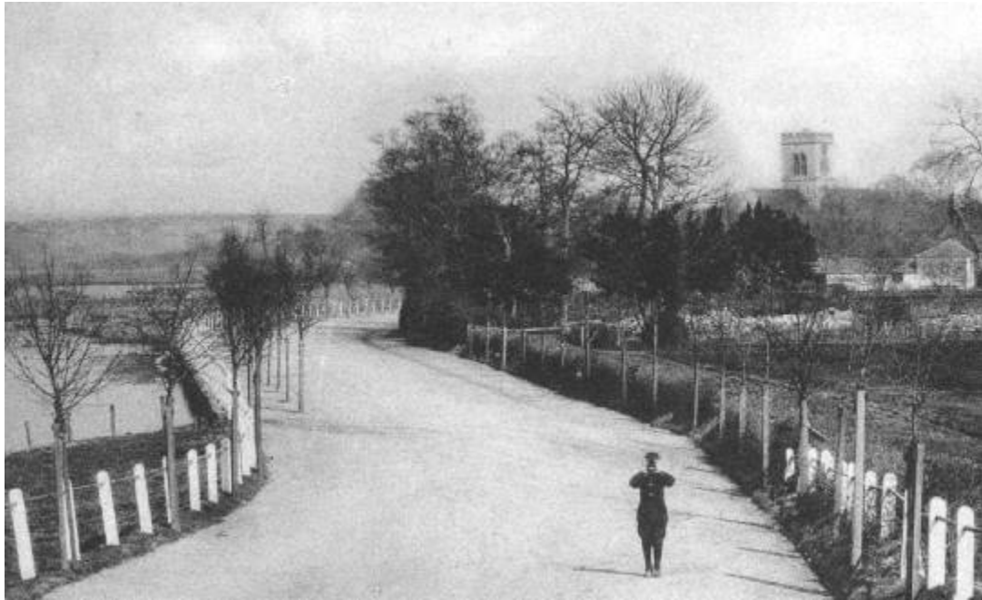
Figure 15. A view from early in the C20th from the King Stream Bridge towards Ringwood. The “Lake” is clearly visible to the left of the causeway, with reed beds projecting well out into it.
