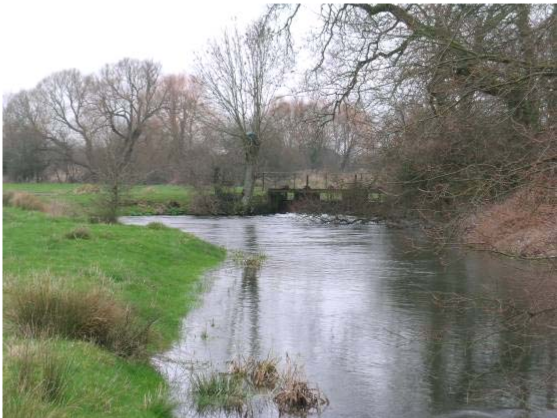
Figure 6.13. Looking upstream to the hatch where the Ellingham watermeadow system leaves the main river in Channel 6.5.
