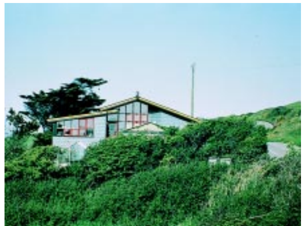
Design solutions should not merely copy the past. This cottage, on the site of a derelict coastguard's lookout post in Cornwall, clearly demonstrates an awareness of the past tradition but is unmistakably modern.
