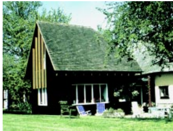
Traditional cottages can be extended to meet changing needs without resorting to standardised solutions.
