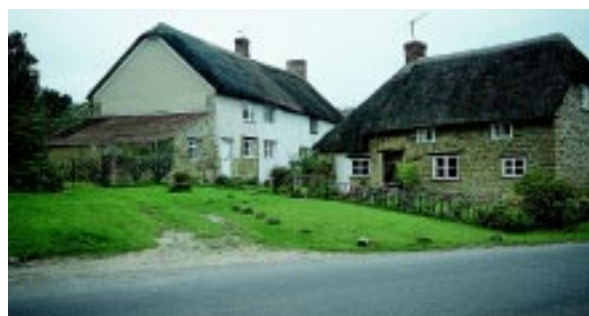
The siting of building in relation to roads and verges is often very locally distinctive. Mells, Somerset.
