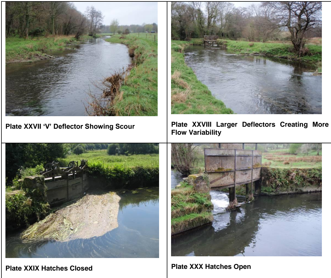
Figure 5.3 Reach 6 Deflectors and Hatch Operations
