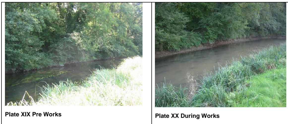
Figure 5.1 Photo Site 36 'V' Deflectors on Left Bank and Brush Clearance
