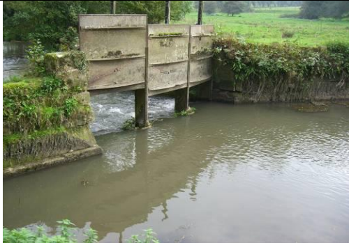
Plate I Sluice Structure at Downstream section of Reach F6
