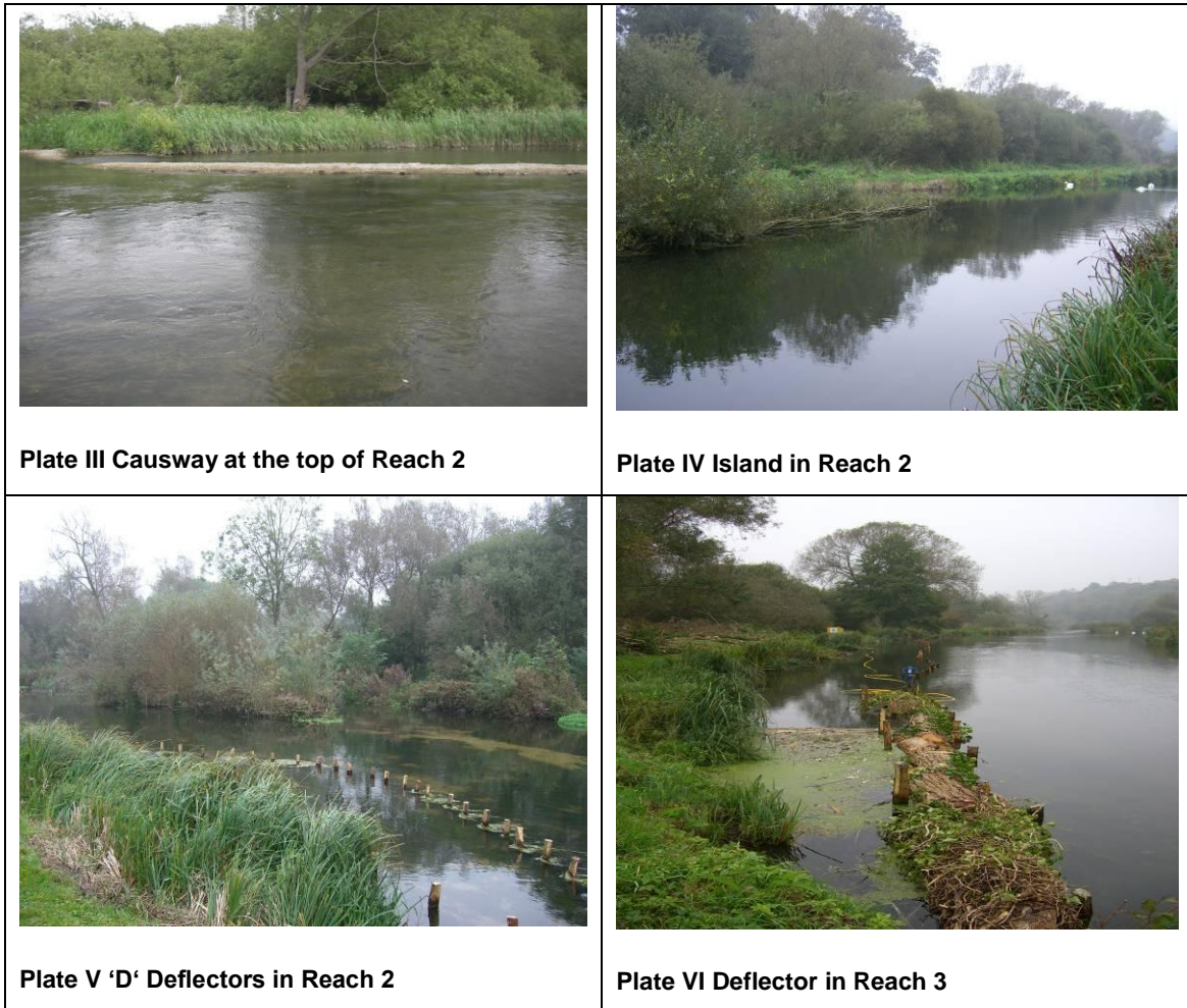
Figure 3.2 Figure 3.3 Restoration structures being built
