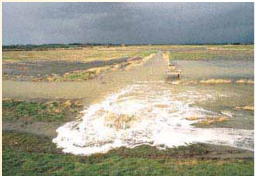
Breaching the sea wall at Tollesbury, Essex.
