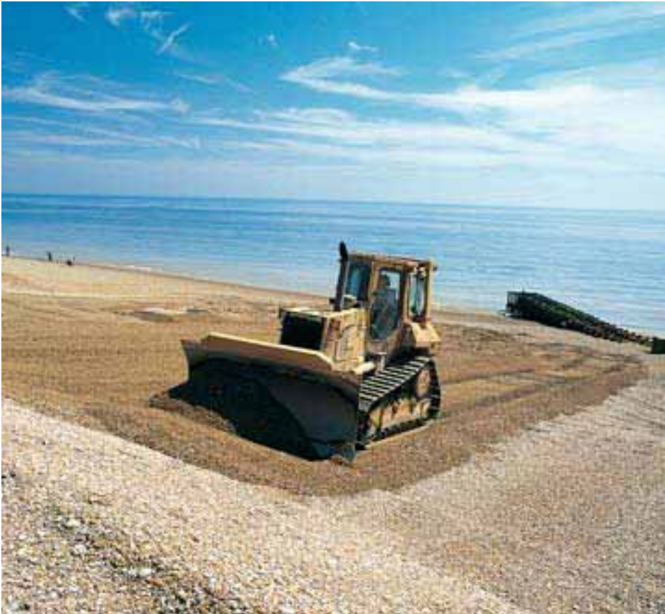
Beach recharge to protect a nuclear power station.
