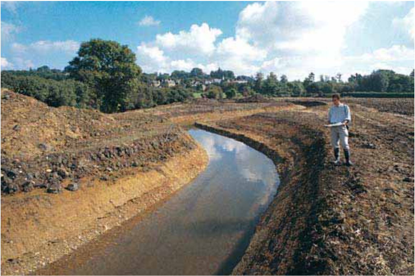
Natural river features being restored on the River Cole, Oxfordshire.
