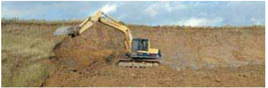
Welton le Wold SSSI, Lincolnshire. Site being restored to favourable condition using heavy machinery.
